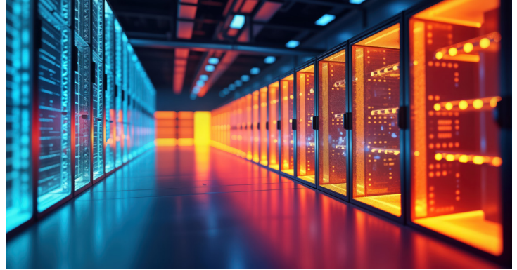
Figure 4: Cooling is one of the biggest engineering challenges for modern data centers. (Source: Maryna/stock.adobe.com)
